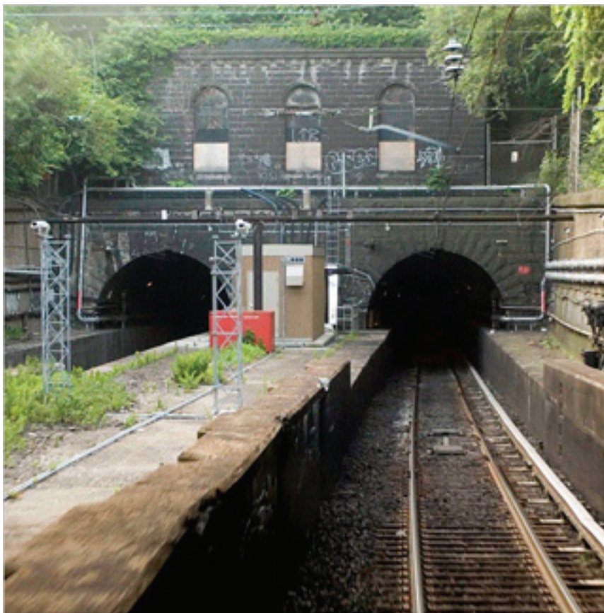
The present tunnel portals used by Amtrak and NJ Transit between New Jersey and Midtown Manhattan.
