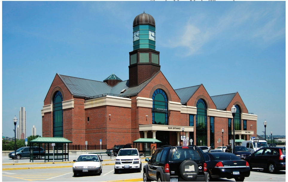
The Rensselaer Amtrak station, now undergoing track and platform work.
