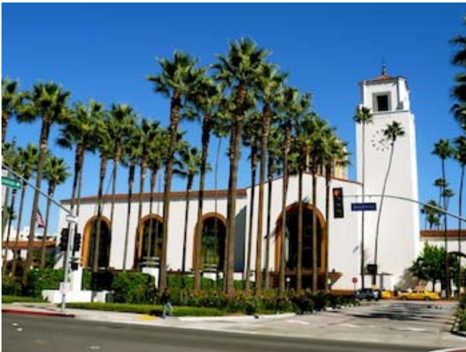
Union Station in Los Angeles
