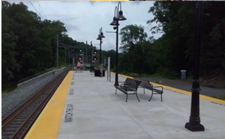
TOP PICTURE, looking northwest, shows car 813 waiting to depart at 4:10 P.M. Sunday, August 21, 2022. To the left of the railing is the wheelchair ramp. A small part of the parking garage is on the right. The open space on the right is where Chester Creek flows under the station. BOTTOM PICTURE, looking southeast, shows the platform, benches, and signals on Sunday, August 21, 2022. The trees on the right side mark the right of way of the Octoraro branch, wiped out in this area by a hurricane in 1972.
