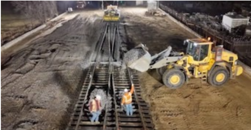
Construction on the Alameda Siding. Photo courtesy of Rio Metro.
